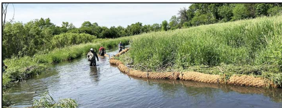
SEWTU VOLUNTEERS INSTALLED BIOLOGS ON WHITEWATER CREEK
