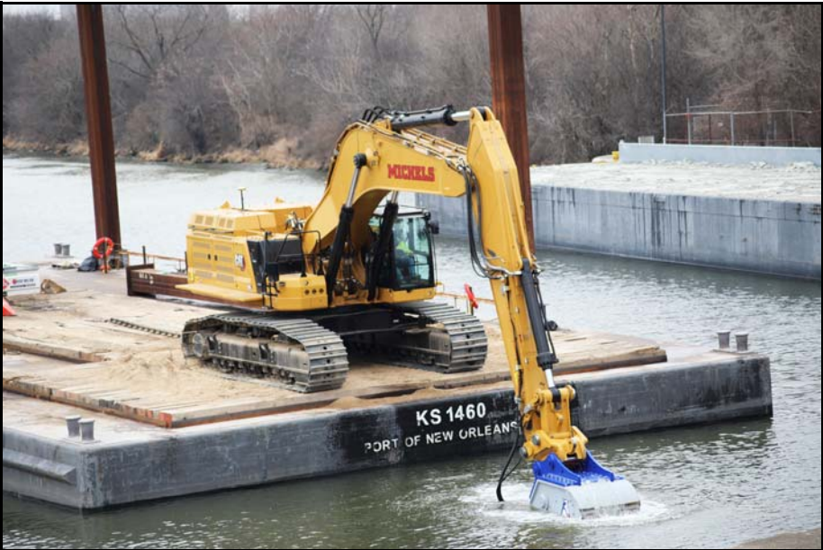
USACE Rock Island District
