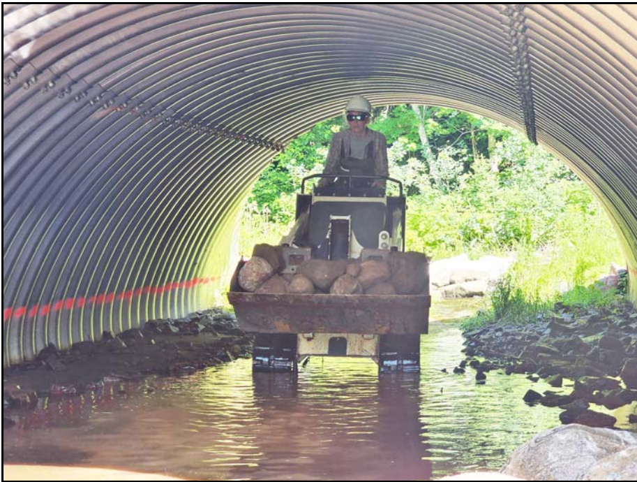
TUNNEL VISION Katti Renik installs stream-bed substrate with the U.S. Forest Service on Whiskey Creek.
