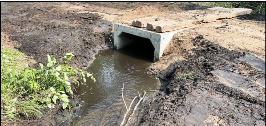
MORE THAN A MILE OF STREAM RECONNECTED WITH NEW BOX CULVERT A new concrete box culvert installed on Chuks Creek in Forest County reconnected more than a mile of trout stream.
