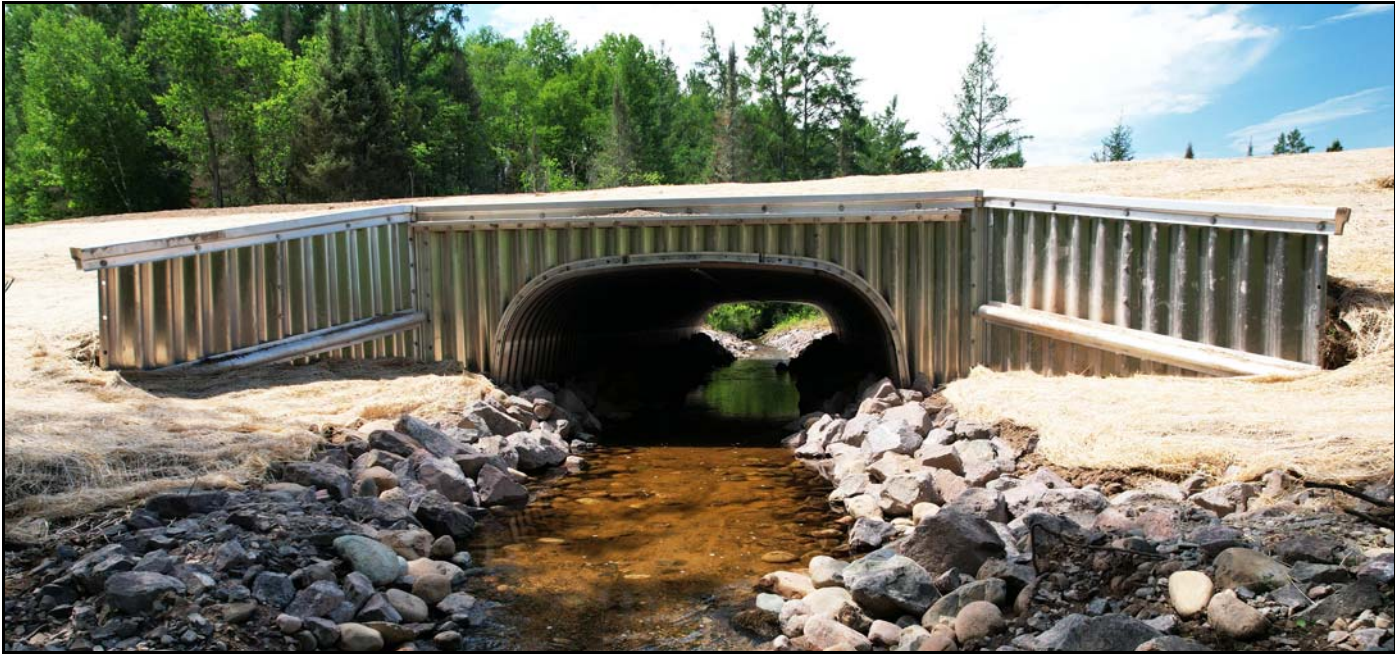
THIS CULVERT ON ELVOY CREEK IN VILAS COUNTY RECONNECTS MORE THAN FOUR MILES OF STREAM
