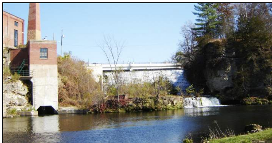
UPPER DAM TO DISAPPEAR, AS WELL AS ITS LOWER COUNTERPART
