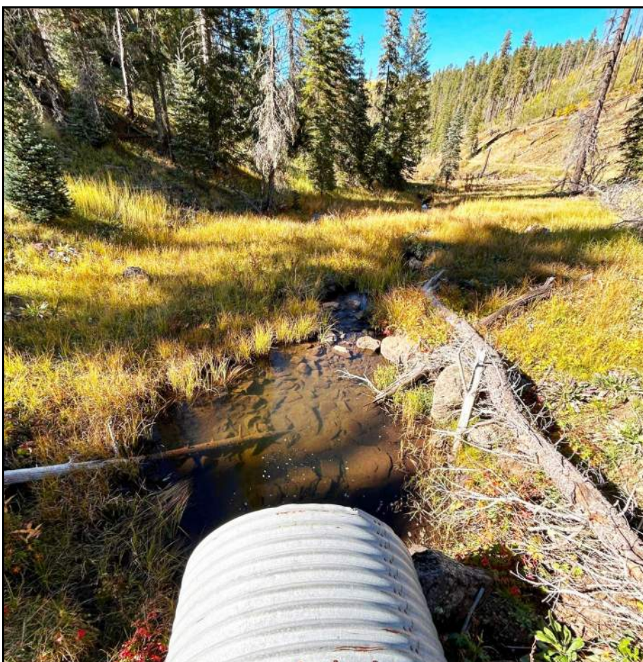
CULVERT POOL ON CORDUROY CREEK
