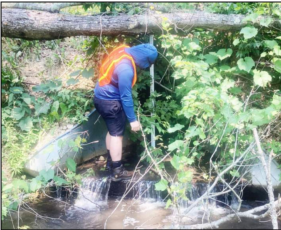
A TECHNICIAN MEASURES A DRIFTLESS AREA CULVERT
