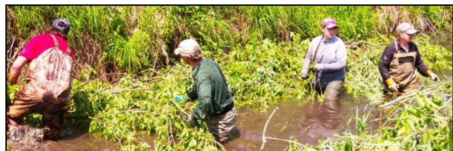
SOUTHERN CHAPTER HONORS DAVE SANDERS WITH WORK DAY Installing brush bundles at SWTU's workday honoring the memory and accomplishments of Dave Sanders.
