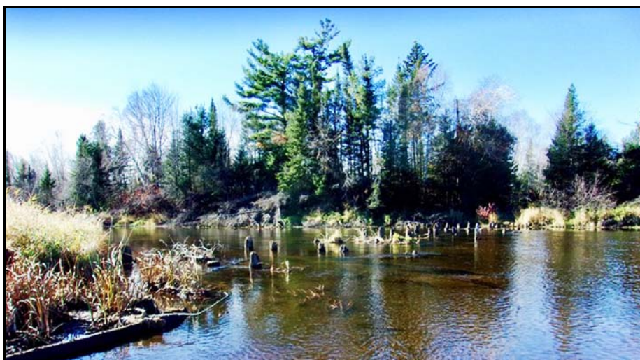
RAILROAD PILINGS STILL IMPEDING FLOW INTO WOLF RIVER The old Wolf River railroad pilings left over from logging days at Pearson, which often catch flotsam and debris.
