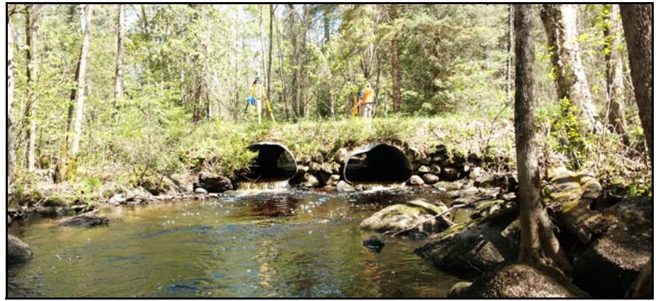
ROCK CREEK BEFORE NEW CROSSING
