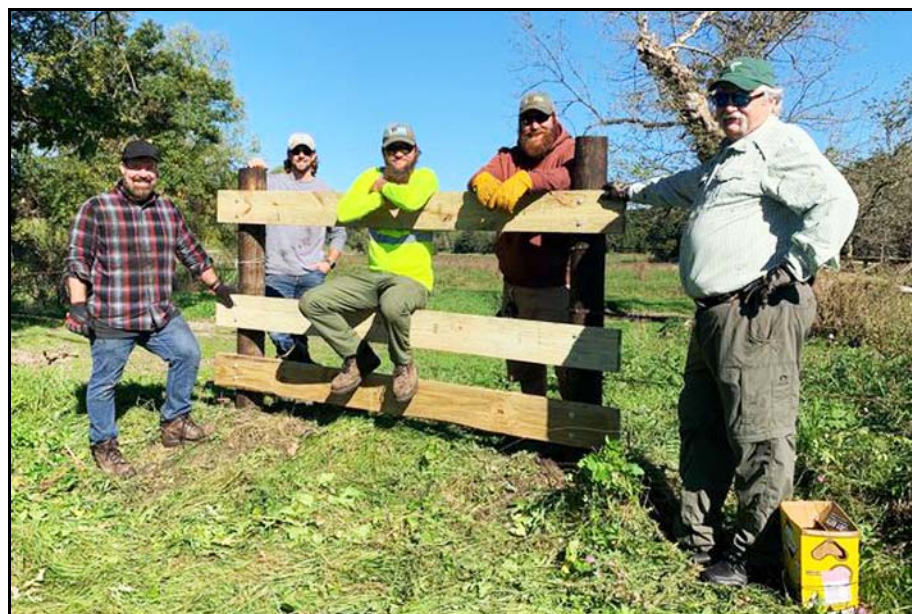
NOHR CHAPTER SPENT SEVERAL WORKDAYS INSTALLING STILES
