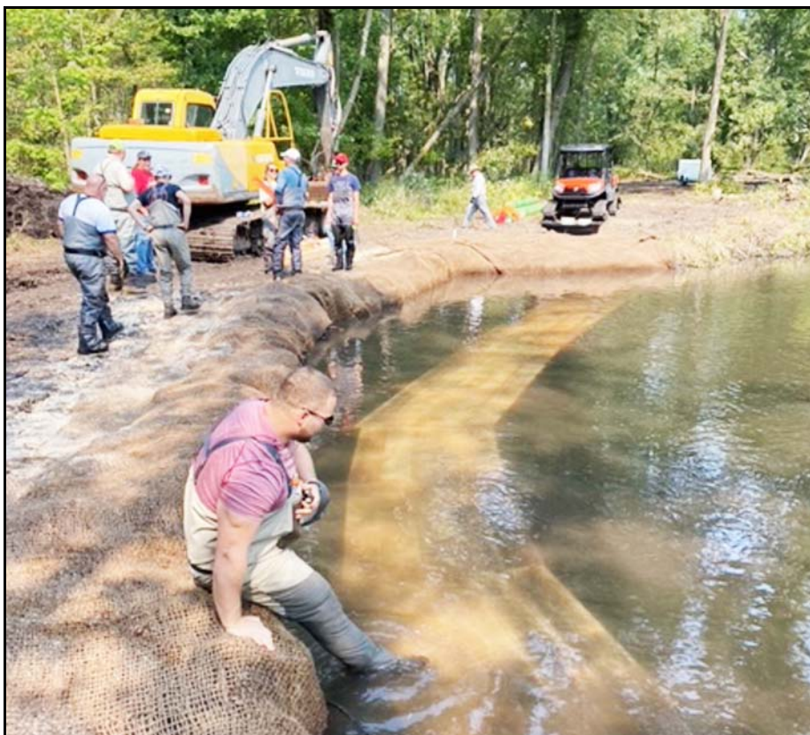
LAKESHORE CHAPTER MAKING GREAT PROGRESS ON ONION RIVER Crews install decking on a bank cover in the Onion River.
