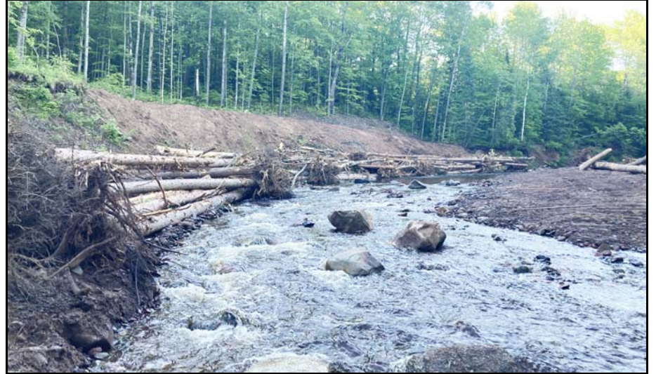
MARENGO RIVER AFTER RECONSTRUCTION PROJECT
