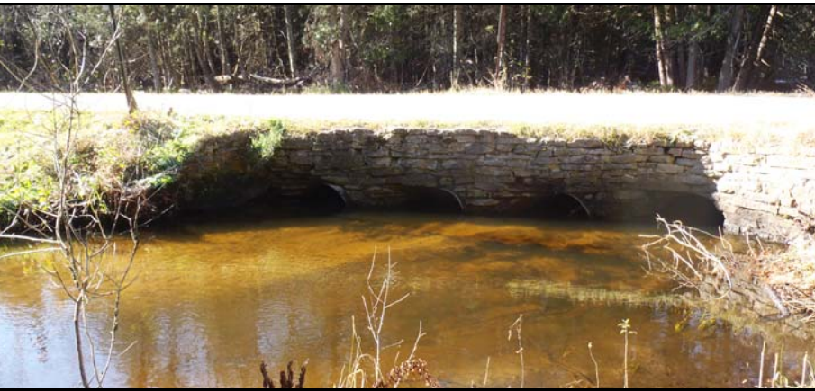
BEFORE: FOUR UNDERSIZED EMBEDDED CULVERTS
