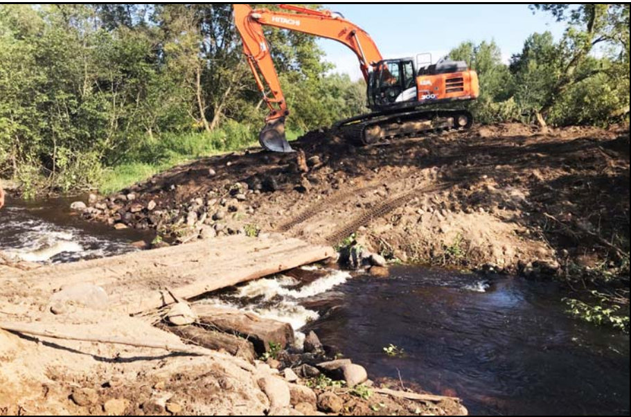
NORTH BRANCH OCONTO RIVER DAM REMOVAL The construction crew from M. Jolma Inc. of Ashland grades stream banks during the remnant logging dam removal.
