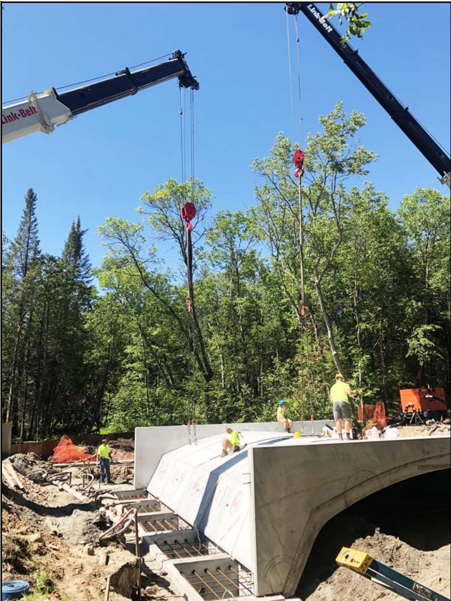
AFTER: PRECAST CONCRETE FOOTERS, FIVE SPANS AND WING WALLS
