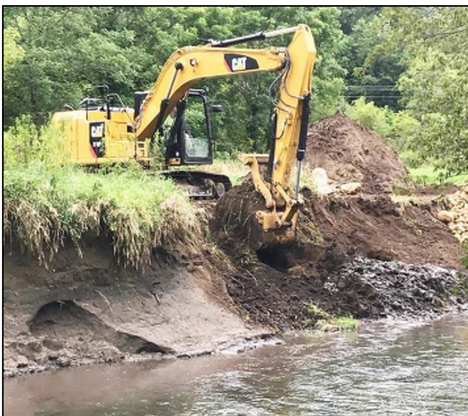
REMOVING A CENTURY'S WORTH OF EROSION ALONG TAINTER CREEK
