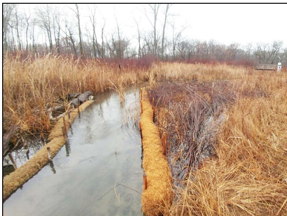
BIOLOGS INSTALLED BY SEWTU ON SCUPPERNONG CREEK
