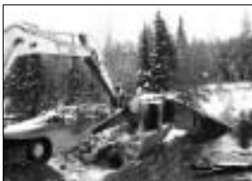
The Woods Creek Dam's eight-foot cement barrier is shown before and during removal in November, 2002.
