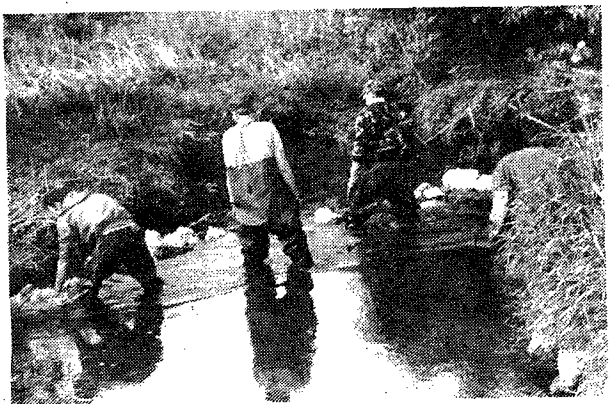
Blackhawk Chapter members at work on Allen Creek Project.
