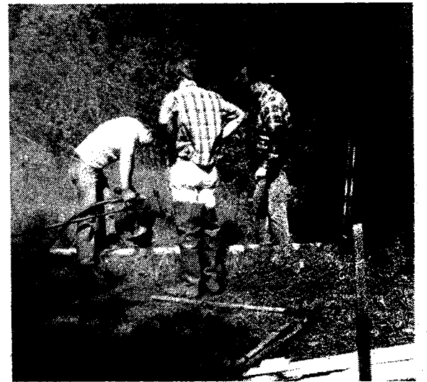
Wally Heil (holding drill), Greg Kornely of DNR, and Darrell Huff labor to install corner posts on South Branch Oconto River project.
