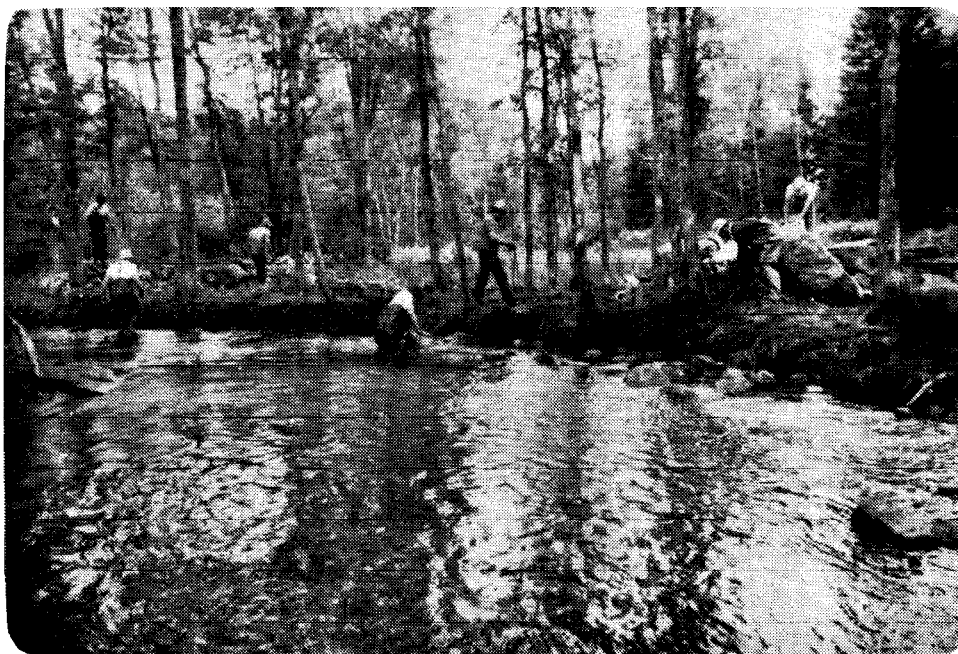
Green Bay TU'ers construct bank cover on Oconto R.
