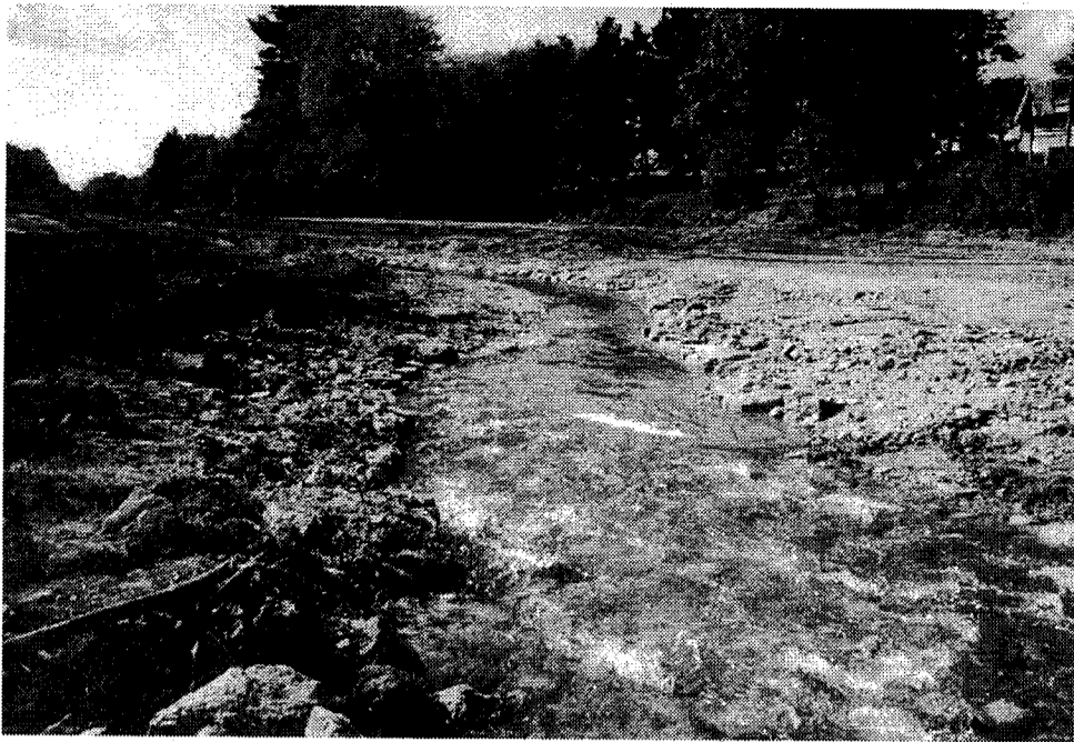
18-Mile Creek above former Colfax Dam before...
