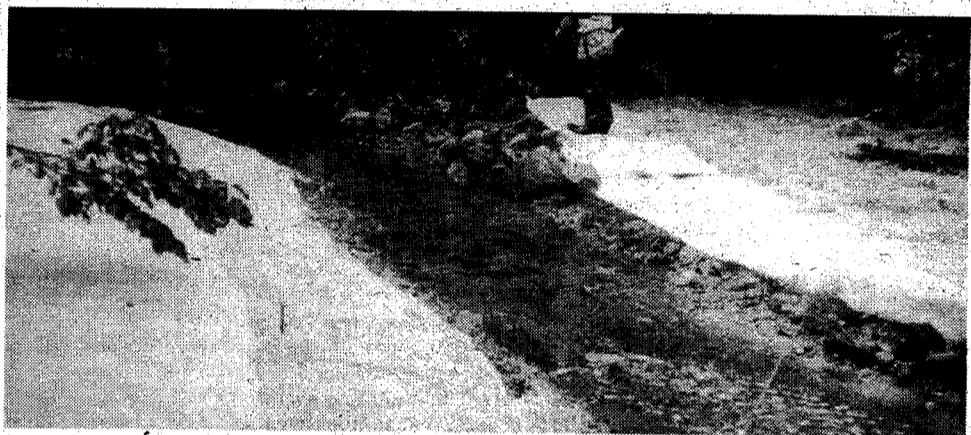
Spring Creek, important feeder to the Elk River, was damaged by Forest Road 517.
