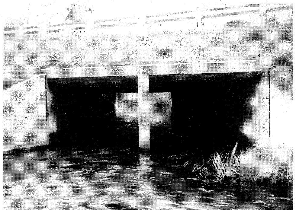
Well-designed concrete culverts on First South Branch Oconto River at Hwy. 32 crossing allow good stream flow, room for high water events and good fish passage.
