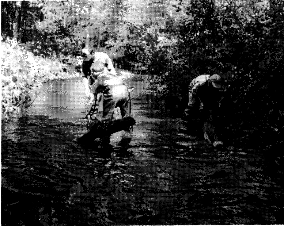
Central Wisconsin T.U. chapter members placing deflectors in Caves Creek.
