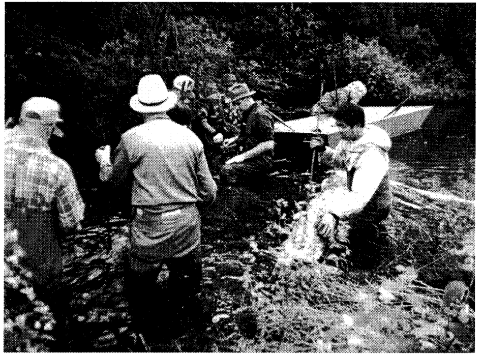
Wisconsin River Valley T.U.'ers install half-logs into the Plover River.
