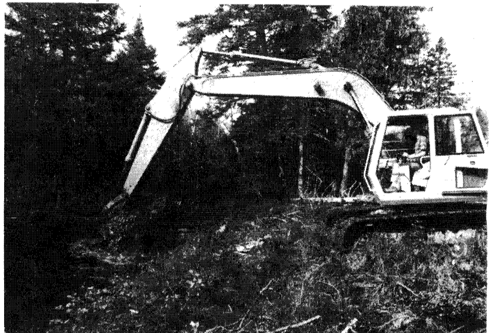
Sediment trap construction on North Fork Thunder River (Oconto County) in 1992.
