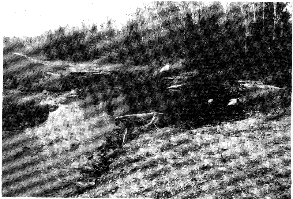
Area of pipeline crossing on North Fork Thunder River to be restored in 1993.
