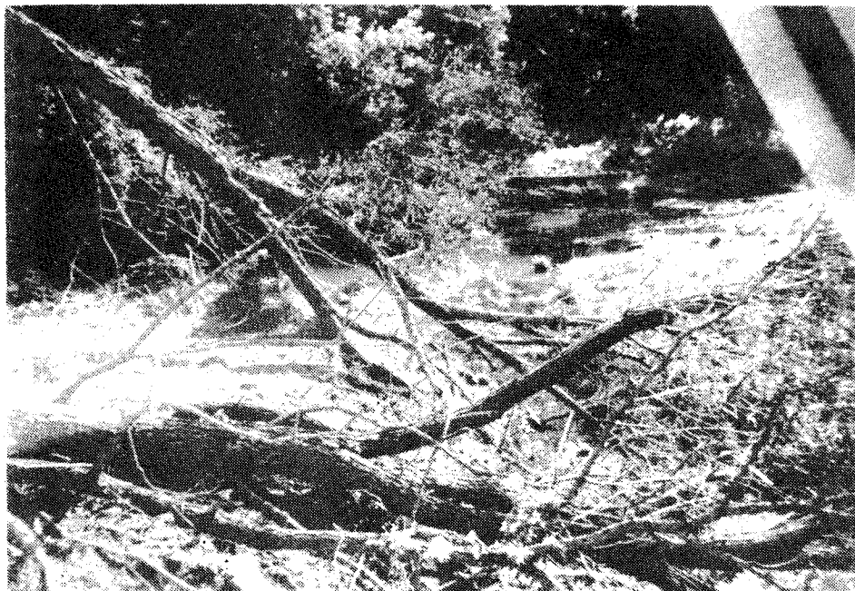
Before - during - after photos of work done on Parker Spring section of West Fork Kickapoo River project in Vernon County, funded by Wisconsin T.U. via a Heilemann grant.
