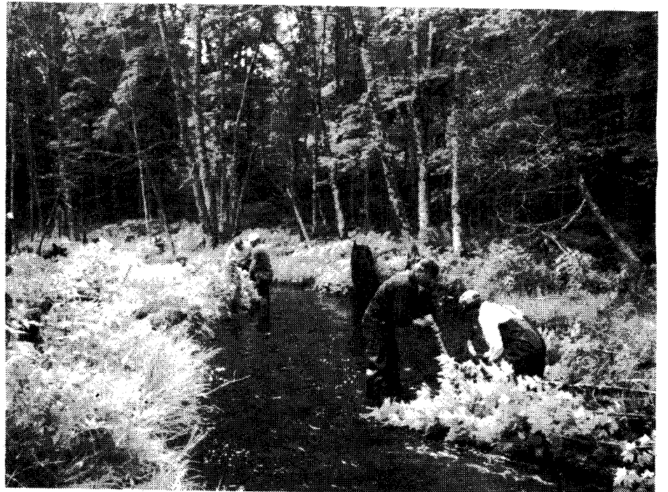
Green Bay T.U.'ers install brush bundles on South Otter Creek in Forest County.
