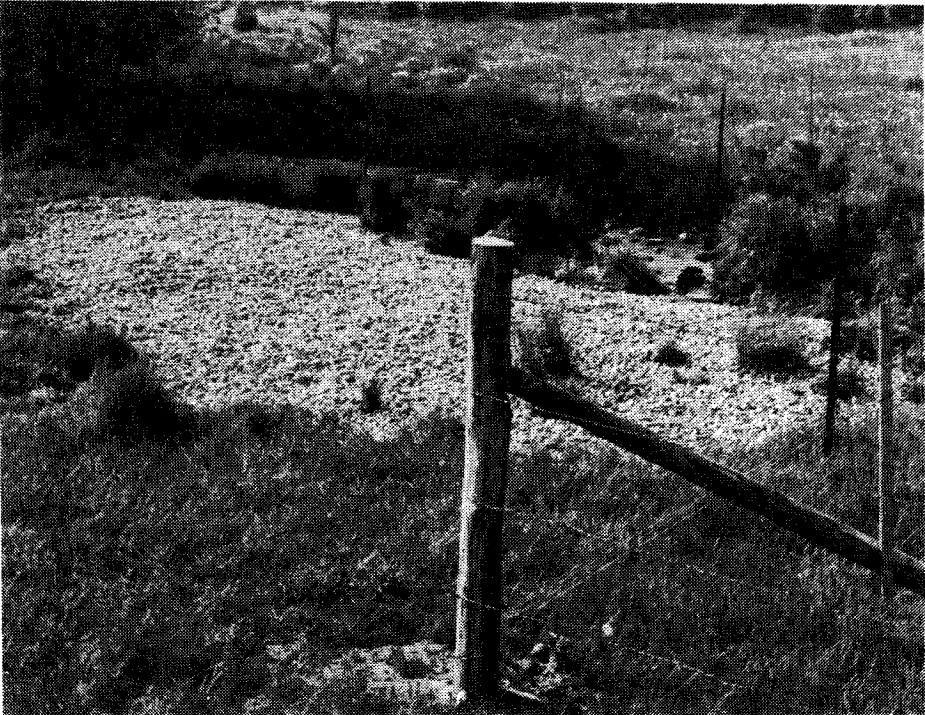
Finished cattle watering station.
