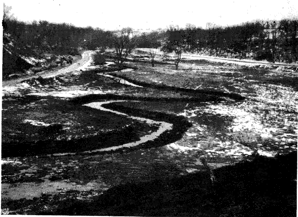
Re-routed section of Brewery Creek nearing completion. Old stream channel is on opposite side of road next to roaster pile at right left.
