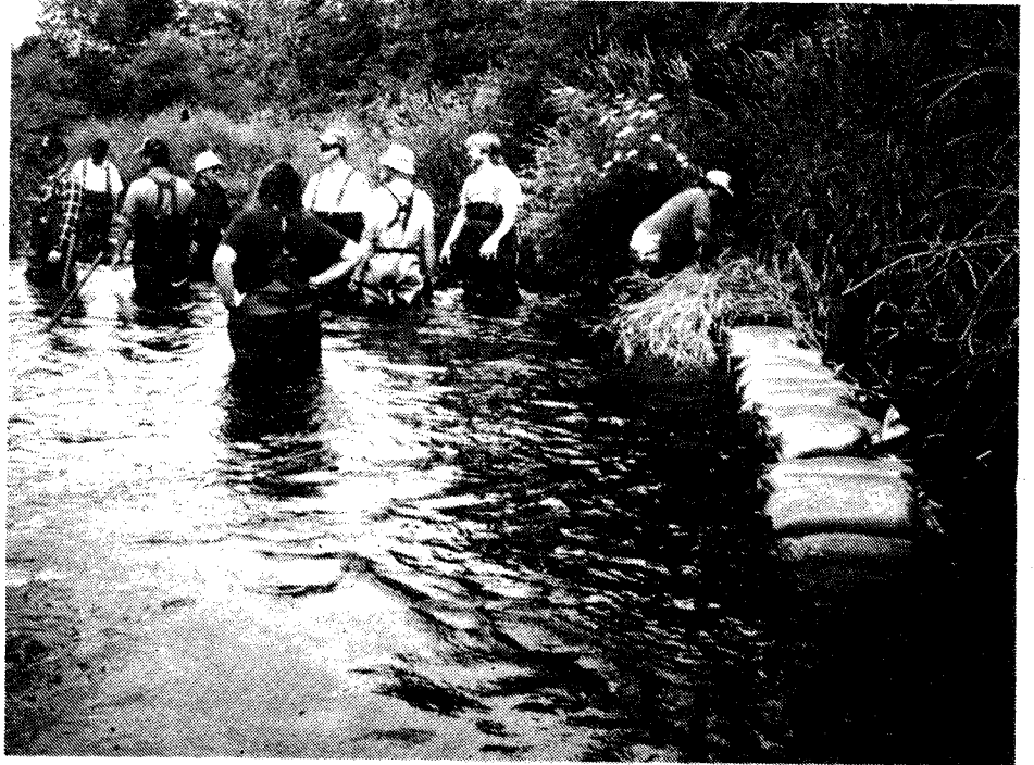
T.U. members from Central Wisconsin and Frank Hornberg chapters apply sod to wing dam on Tomorrow River below Nelsonville.
