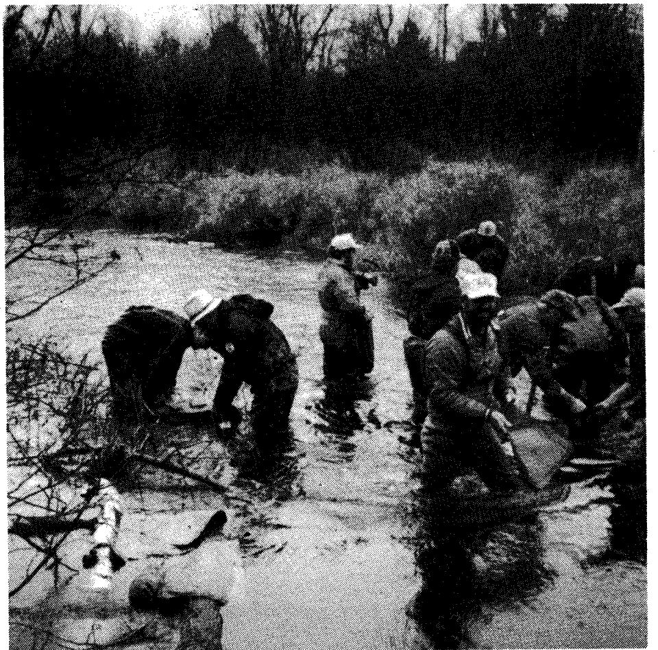
Central Wisconsin TU'ers place sand bags inside bank deflectors in the Tomorrow River to wash sediment out of stream.
