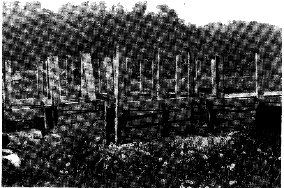
"LUNKER" structures waiting to be installed in West Fork section.
