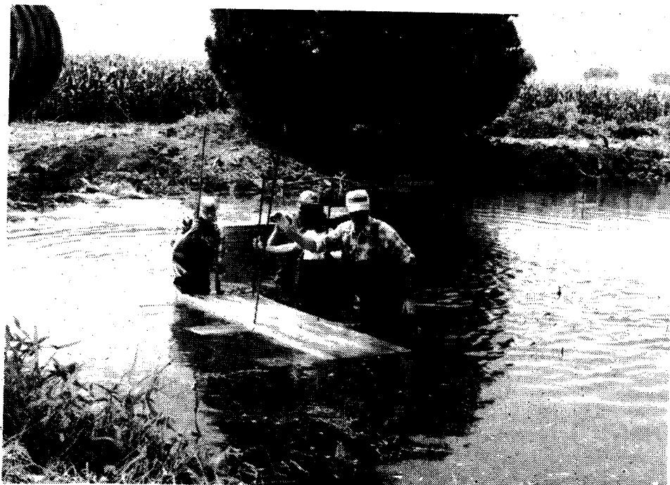
Southern Wisconsin T.U.'ers install "lunker" structure in Black Earth Creek (Dane County).
