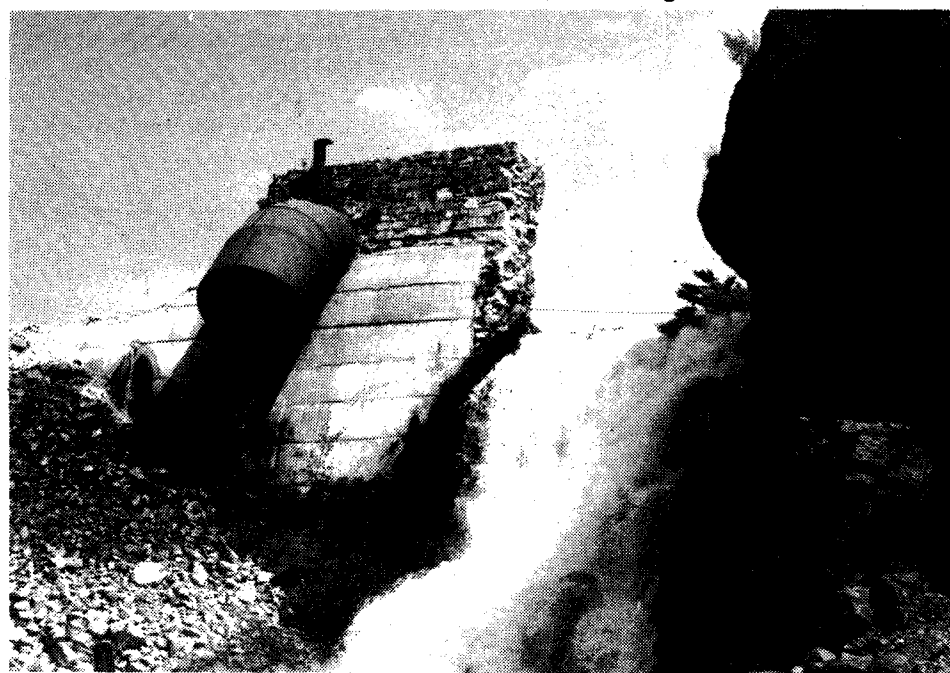
Breaching of Prairie Dells Dam is allowing Prairie River to return to its former streambed.
