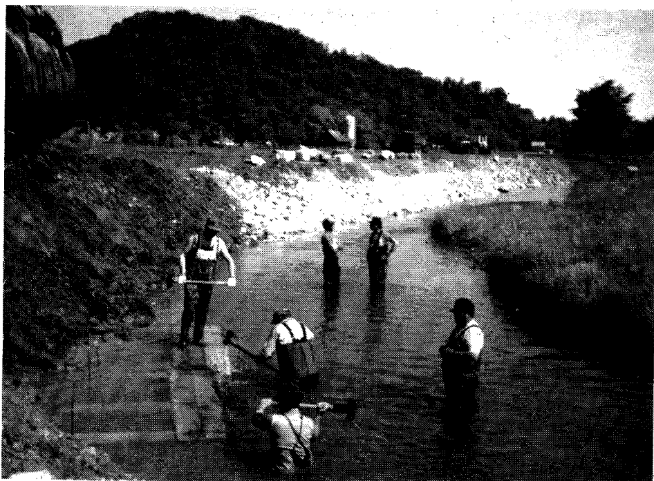
Blackhawk T.U.'ers install a "lunker" structure in the West Fork Kickapoo River (Vernon County).
