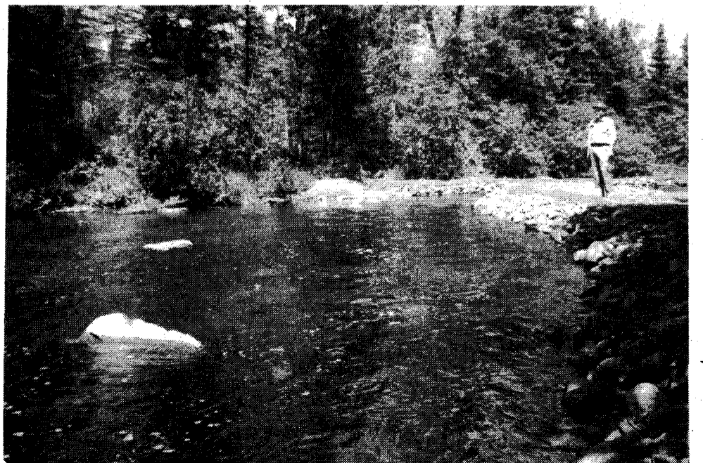
A section of the S. Branch of the Paint River after completion of work is shown.
