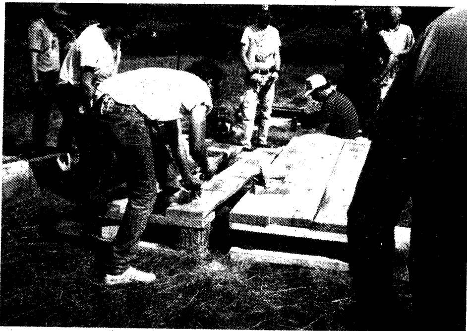
Southern Wisconsin T.U. chapter members build "lunker structures" for Zander farm project on Black Earth Creek.
